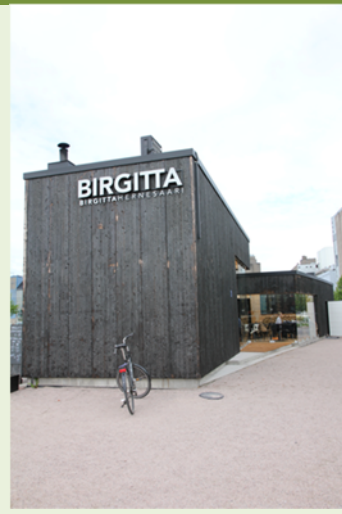
Café Birgitta , Hernesaari, Helsinki 2014. Talli Architecture and Design. A modern log building with a façade combined with charred wooden surface and large glass windows opening a sea view. Design by Architect SAFA (Finnish Association of Architects) Minna Lukander, and the logs provided by Honkarakenne.
